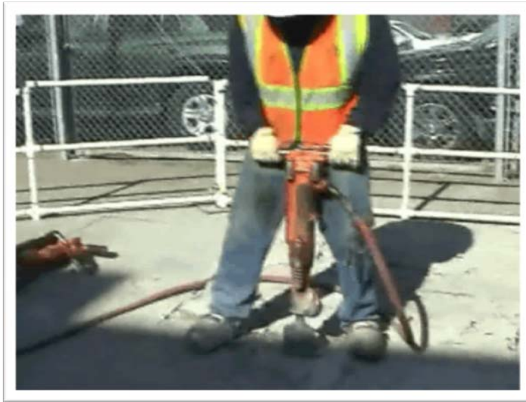
Figure 1: Worker using traditional jackhammer
