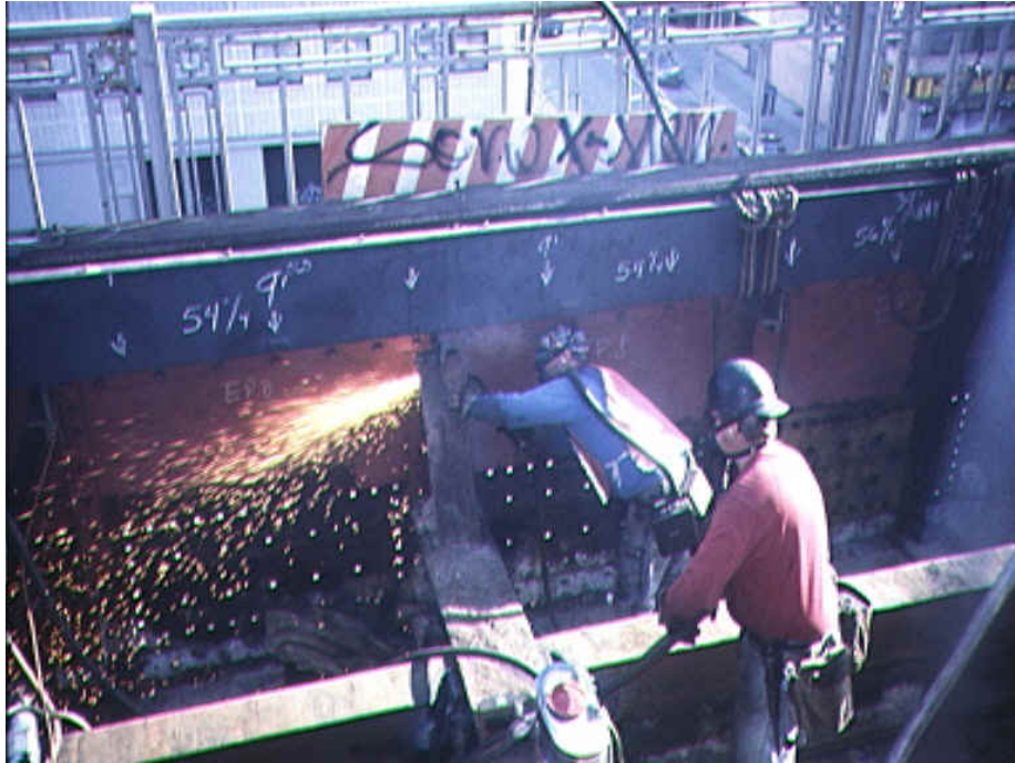
Ironworkers rehabilitating a steel bridge (could fall under 16XX or 17XX steel erection)
