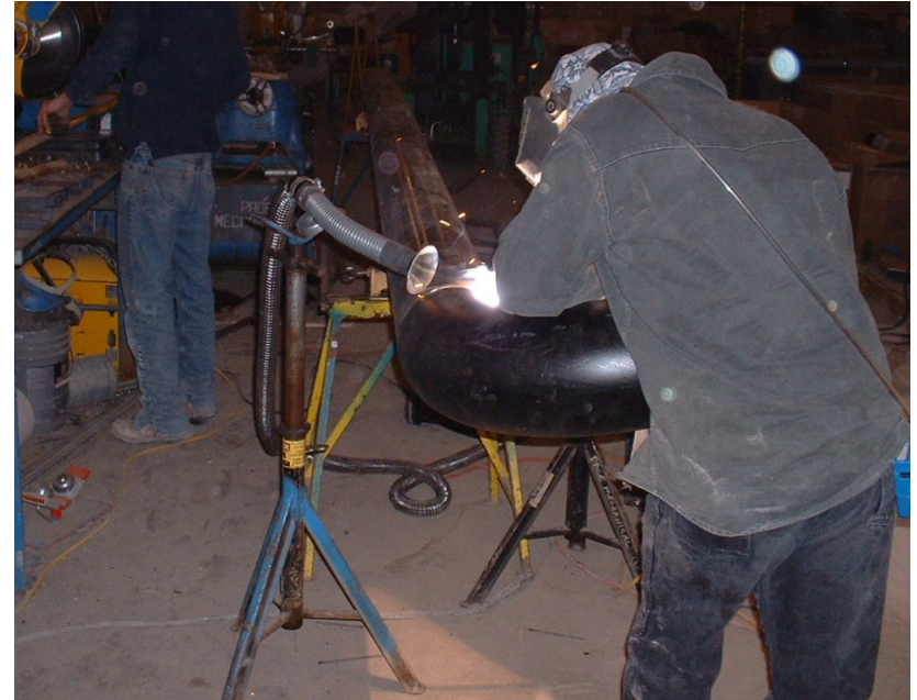
Pipe-fitter/welder working on HVAC piping during new construction of a university building
