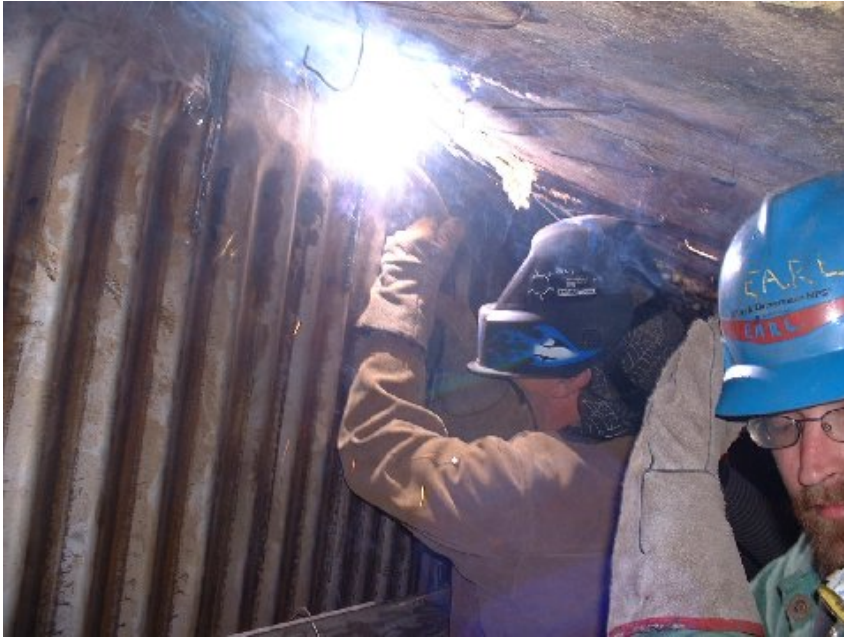
Boilermakers work on boiler tubes during power plant rehab/maintenance
