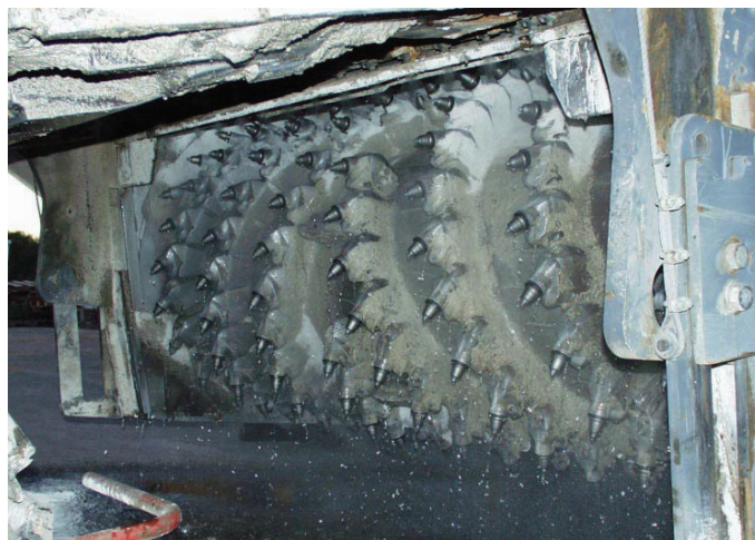
Figure 3. Water application at drum to cool cutting bits. The water is then mixed with asphalt pavement material as it is removed by the cutter bits (Photo by NIOSH)
