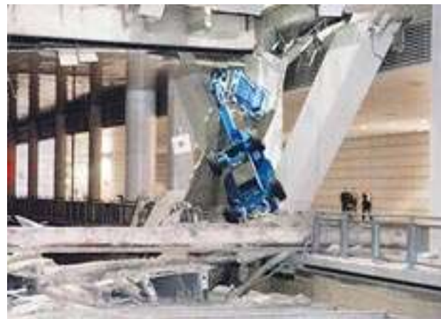
Figure 2 Structural collapse from weight of equipment
