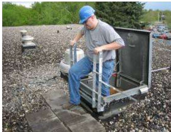
This photo shows horizontal grab bars
