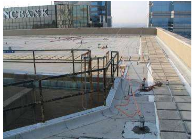
This photo shows guardrails installed along an opening. Installing guardrails early on in the construction process can eliminate the risk of a fall through an opening.
