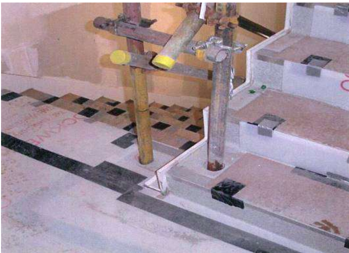
This photo shows cast sockets along the open side of a stairway. The sockets make it convenient to install temporary or permanent guardrails.
