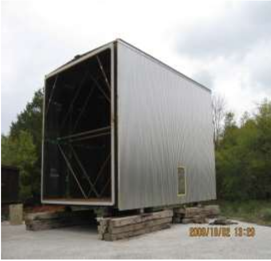
Figure 3- Insulated before raising into place
