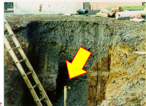
Watch for impalement hazards at base
