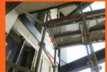
SEPTEMBER Interior rough-in continues
