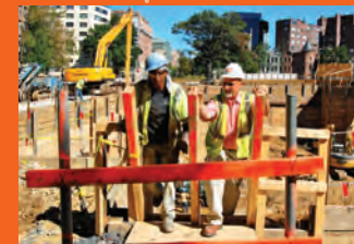
AUGUST Early construction: Sheeting and shoring process
