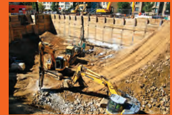
JULY Early construction: Creating basement levels
