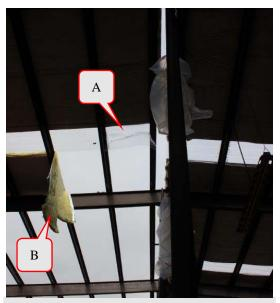
**Figure 5.** Skylight that collapsed under the roofer (A); insulation that tore (B).
