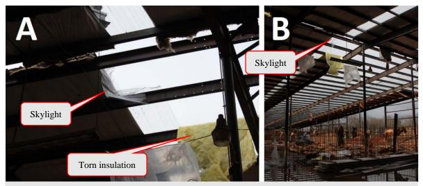
Figure 3. Skylight through which the victim fell with torn insulation (A); interior of the building (B).
