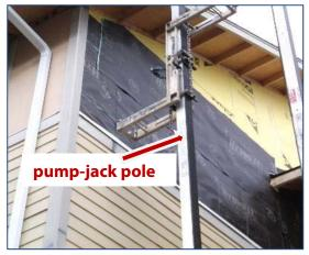
Figure 1 (above). Breezeway, pump jack pole. Figure 2 (below). Breezeway, 3<sup>rd</sup> floor stair landing with temporary railing.
