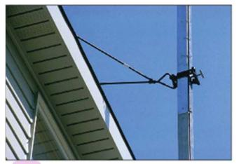
Figure 5. Example of scaffold pole properly secured to building (from OR-OSHA publication, "Supported Scaffolds").
