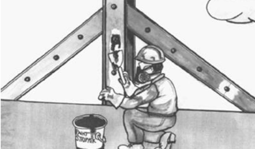
Stripper is applied to steel surface and left in place for 1-24 hours. Paint and stripper are scraped off and residues are wiped away. Some strippers require neutralization.
