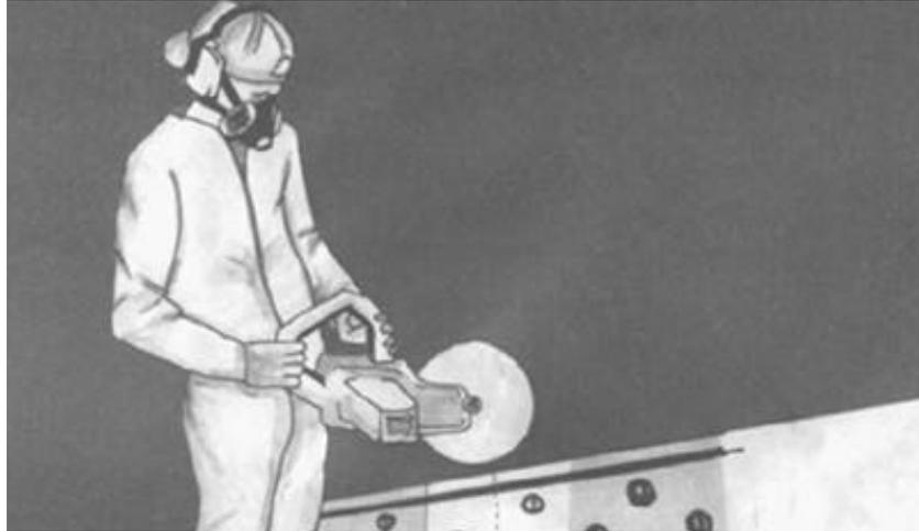
**Mechanical removal** of steel is an alternative to torch cutting. Steel members are disassembled by reversing installation procedures - removing rivets and bolts first and then uninstalling steel beams. Also, chop saws, hydraulic shears, or metal cutters can be used.
