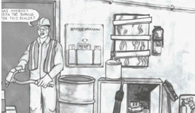
Lead paint is removed with power tools equipped with dust collectors prior to other lead-emitting activities. Small lead particles are collected by a HEPA vacuum system as they are released by the tools.
