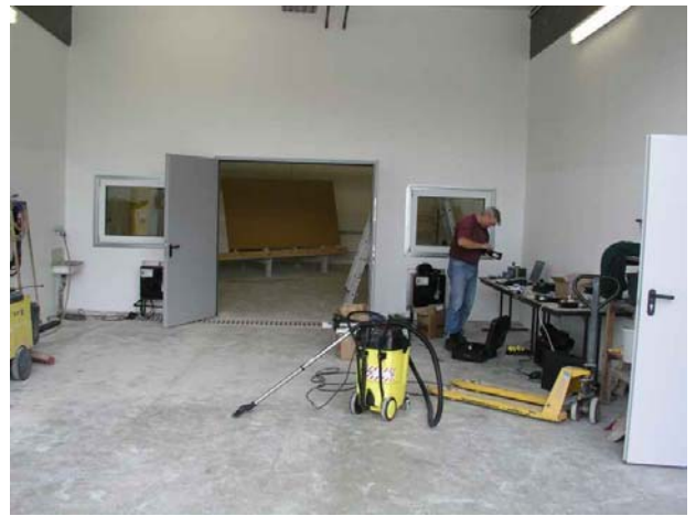
fig. 5.3 - 3 Hall 17 after its transformation with vestibule in the front, test room in the back
