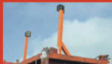
»» These protruding legs could easily become entangled with the lifting gear causing a hazard to those involved in loading or offloading.
