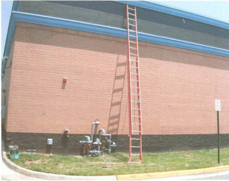
Ladder collapsed – worker was able to grab on to the leading edge of the building
