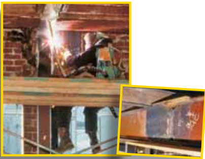
Strip back paint before cutting or welding.
