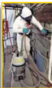
Attach power tools to a HEPA vacuum.
