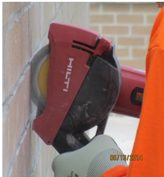
Figure 5. Hilti grinder and Dust Guard
