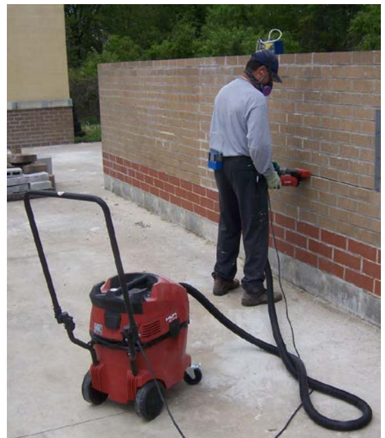
Figure 3. Hilti grinder with Dust Guard and VC40-U vacuum
