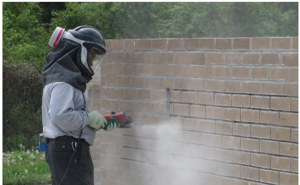
Figure 1. Hilti grinder without tuckpointing LEV system
