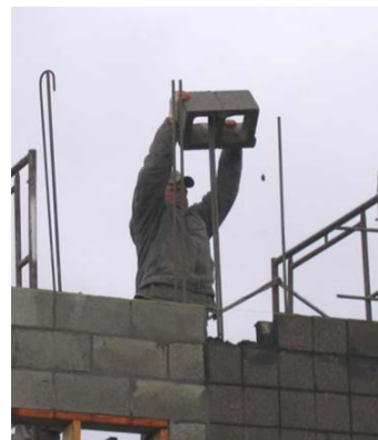
Laying CMU over rebar
